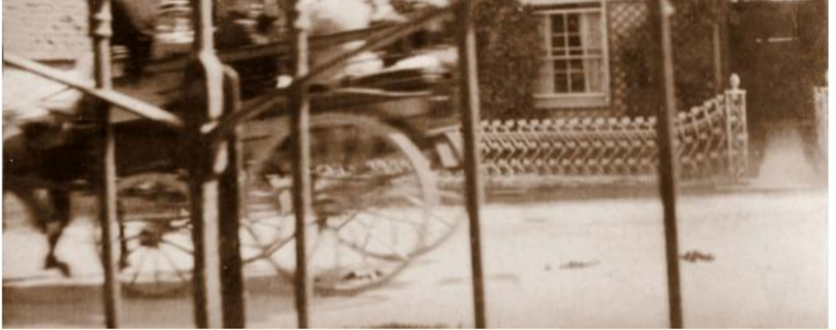
A carriage speeds past Sanford House. The building was demolished in 1958 to improve access to Lower Sea Lane. To the left can be seen the workshops of Pryers, the Stone Mason and Builders, which is now the Pharmacy shop.
