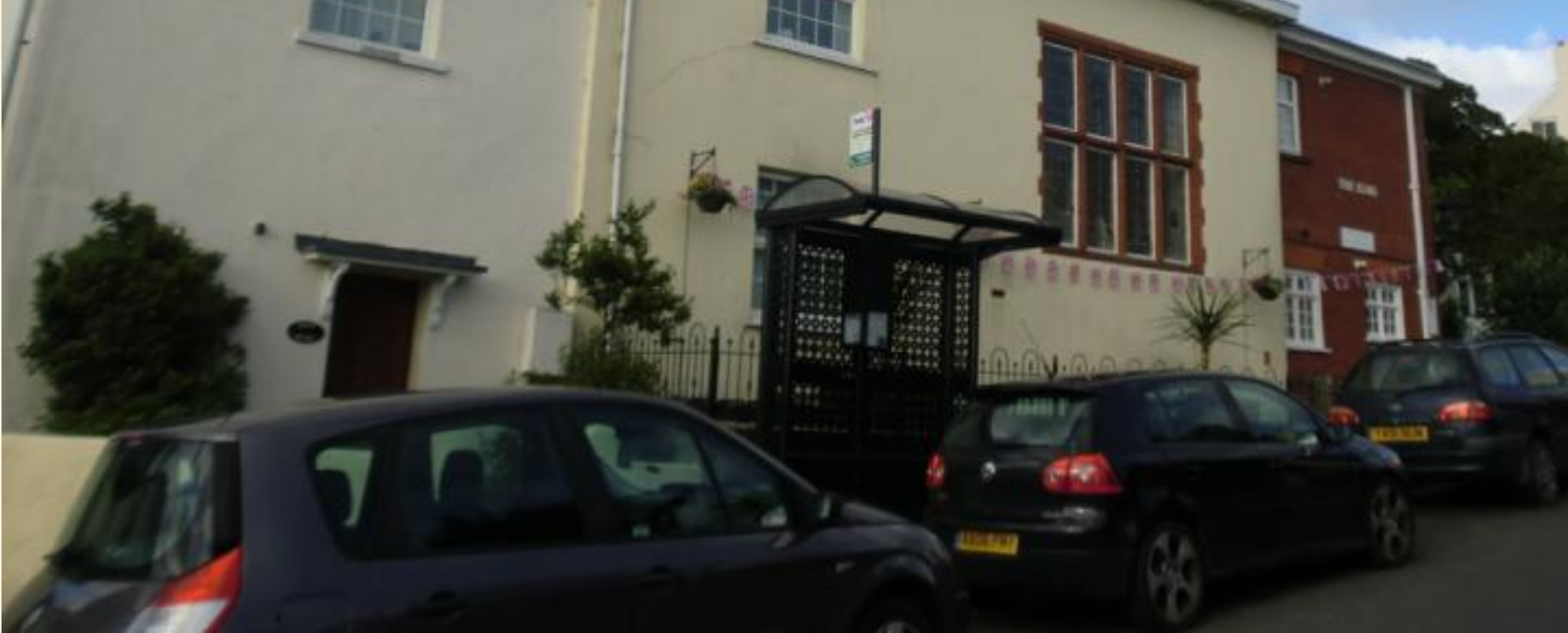
The Elms was dramatically altered and enlarged by Dr Norris in 1920 as can be seen by comparing the previous photo with today's.
